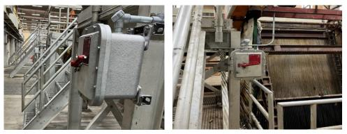
New local disconnects installed for the bar racks at Pump Station 2  $\,$
