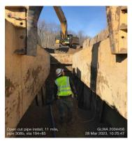
Trenches for open cut pipe installation
