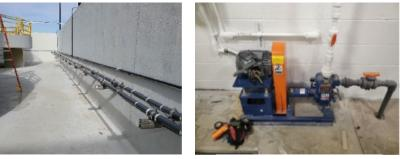
Heat-Traced Ferric Chloride Piping
