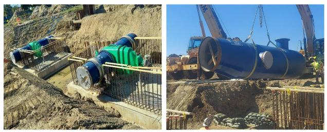
48" Gate Valves installed in vaults V-16 and V-17 with vault construction underway
