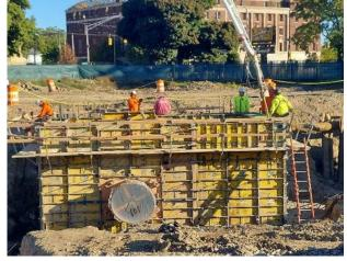
Crews pouring concrete for the reinforced walls at vault V-14
