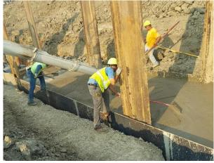
Pouring controlled low-strength material around installed steel pipe
