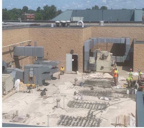
Overview of concrete removal and patching above Ozone Contractor #1
