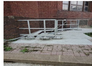
Task 2J-01 Upper Wet Well Stairwell
