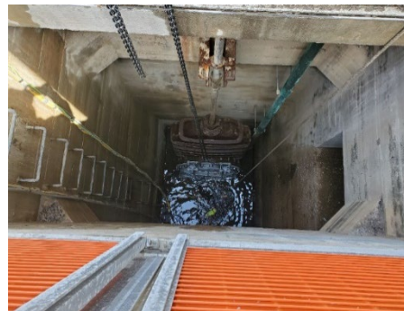
Flap gate being installed
