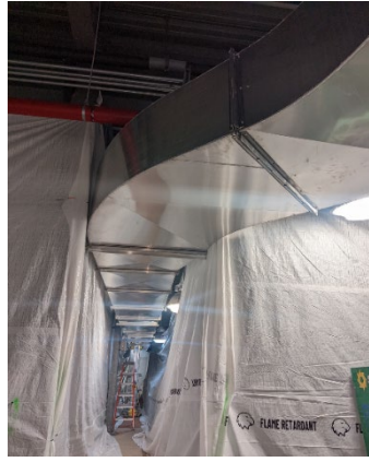
Newly installed ductwork in sedimentation area
