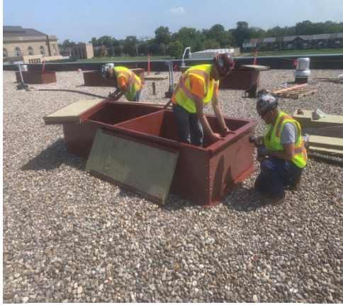
Assembling and installing roof top curbs for new HVAC units
