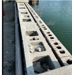
Capstones repairs at CON
