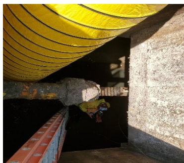
Surge Basin After Second Chemical Cleaning
