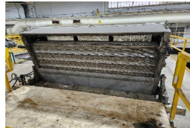
Screen #8 is being rehabilitated
