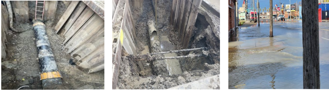
24-inch watermain break at Harper and Hayes
