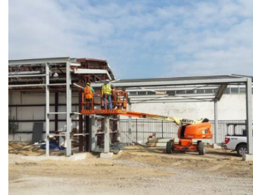
HAZMAT – Steel Structure
