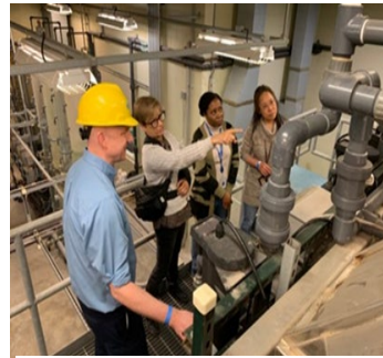
Waterworks Park Pilot Plant
