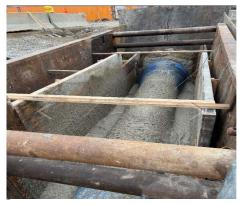
42" to 60" Connection and controlled low strength material (CLSM) Encasement
