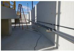
Damaged Ferric Chloride discharge piping is replaced by the Contractor shown above
