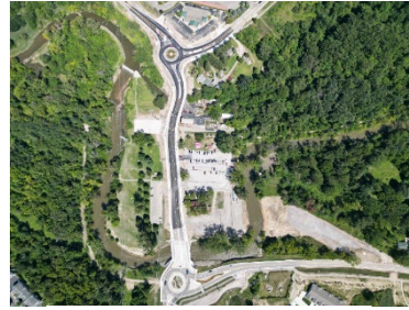
Aerial photo of completed roadway improvements
