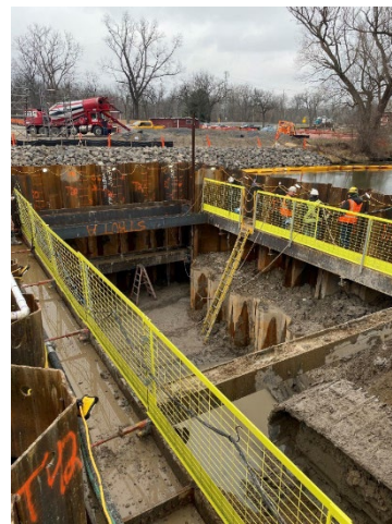
Stage 1 of cofferdam installation within the Clinton River
