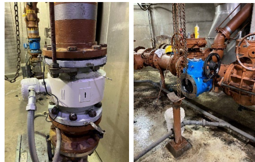
New ABB flowmeter installed and 8" plug valve installed for Sludge Pump 22
