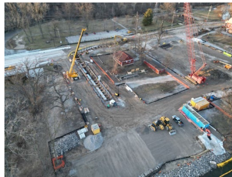
WTM installation entering Avon Rd near the Avon/Dequindre roundabout
