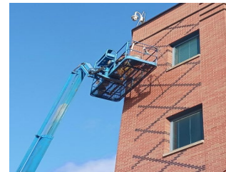
Caulking replacement at NAB.
