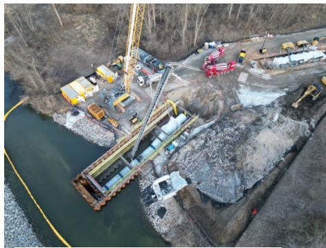
Installation of WTM within Stage 1 of the cofferdam system
