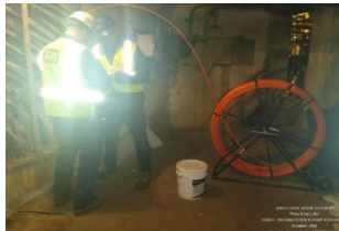
Existing Conduit Investigation
