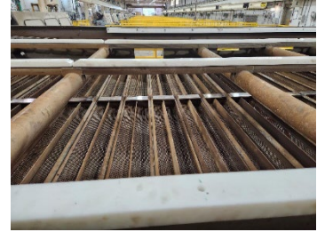
Screen # 15 is being rehabilitated
