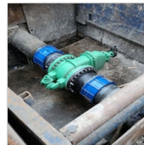
Photographs show the installation of the new valve
