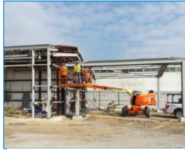
HAZMAT – Steel Structure
