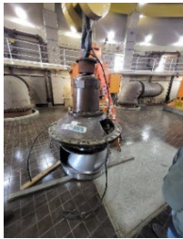
RSP 13 pull-out assembly ready for loading
