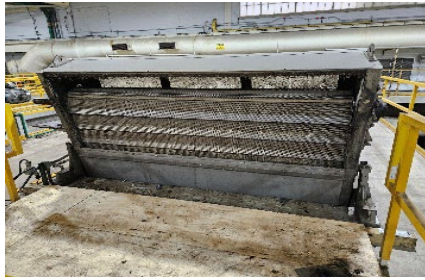
Screen # 8 is being rehabilitated
