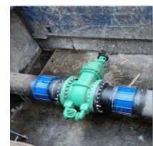
Photographs show the installation of the new valve
