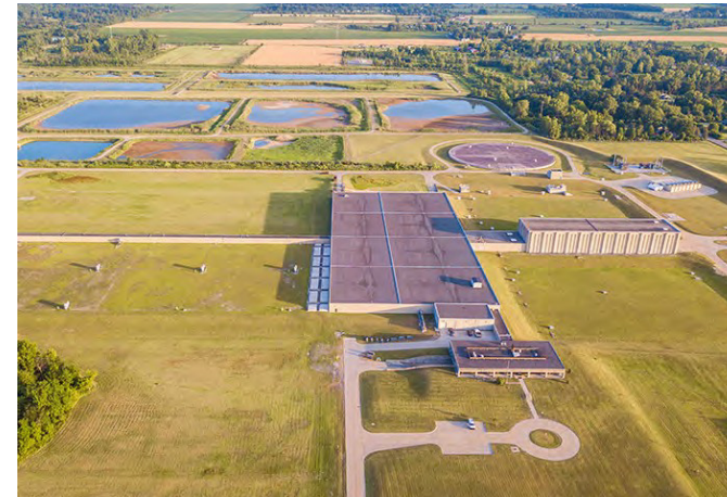
Figure 3. Lake Huron WTP
