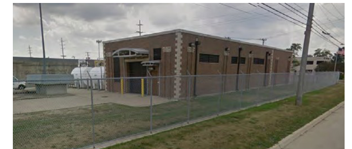
Figure 35. Schoolcraft Pump Station
