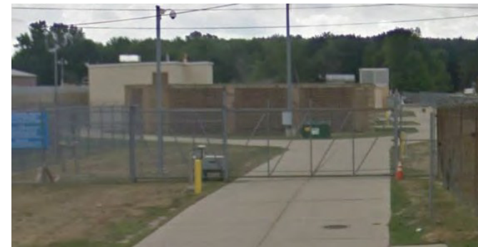
Figure 27. Joy Road Pump Station
