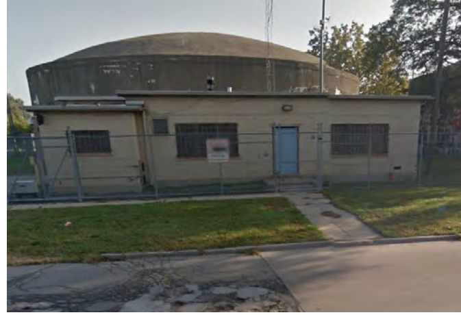
Figure 22. Electric Avenue Pump Station
