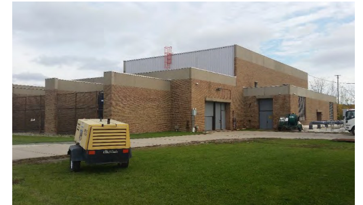
Figure 61. Northeast Pump Station
