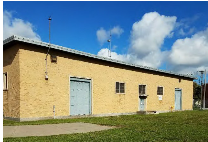
Figure 21. Eastside Pump Station
