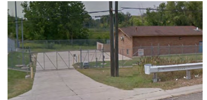
Figure 32. Orion Pump Station
