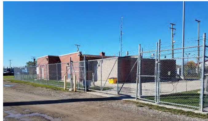
Figure 26: Michigan Avenue Pump Station
