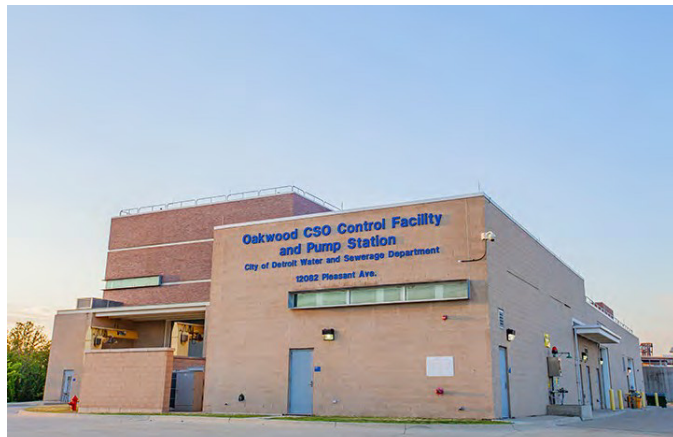
Figure 42. Oakwood CSO RTB
