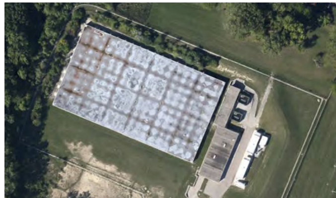
Figure 25. Franklin Pump Station
