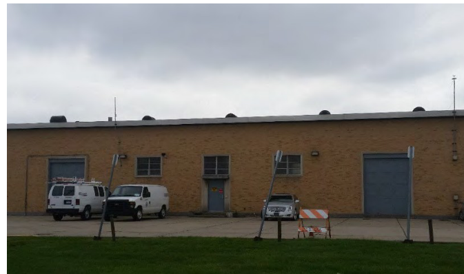
Figure 30: Northwest Pump Station
