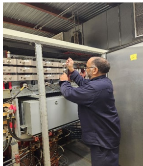
Left: Shane Clarke inspecting one of the eight sanitary motors at Freud Station. He is looking at the slip ring brushes to check for proper seating and length. He will also check for excessive dirt that may be on the rings, brush holders, and insulators, and will then clean them
