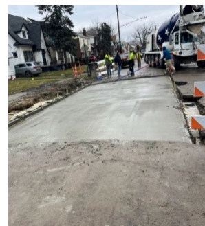
72-inch watermain leak in Detroit: Road restoration
