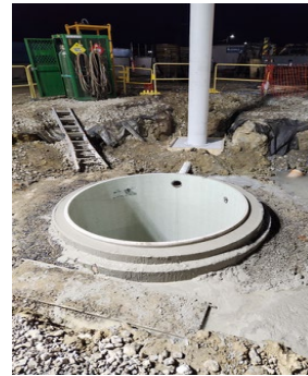
Installed permanent shaft and vent Northeast WTP Raw Water Tunnel
