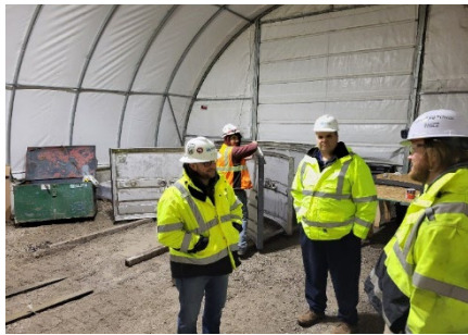
Stainless steel liner plates being staged for installation
