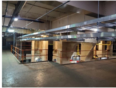
New cable tray installed in Turbine House basement
