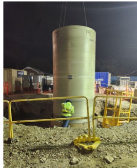
Installation of permanent access shaft Northeast WTP Raw Water Tunnel
