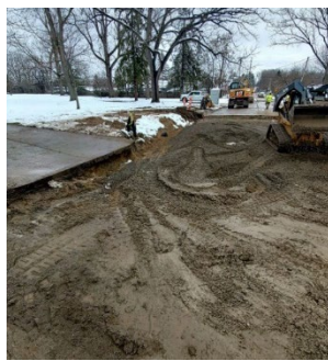
30-inch watermain break in Northville: Road restoration at the break site
