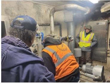
Left: Dave West is inside one our variable frequency drives (VFD) at Imlay Booster Station. EICT-E is working alongside ABB to upgrade these drives so that they will be dependable for years to come
