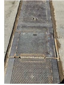
The repaired stop log cover in the street at WRRF
