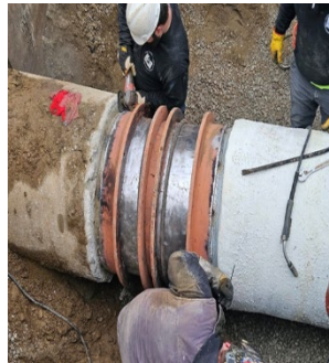
30-inch watermain break in Northville: Installation of repair kit
