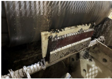
The UHMW wiper modification has improved grit removal effectiveness from grit cross-conveyor
