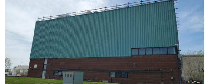
2022 WRRF Roof Improvements Project
