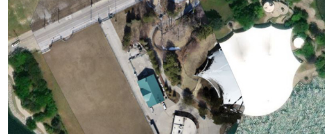
CSO Facilities Improvements II
