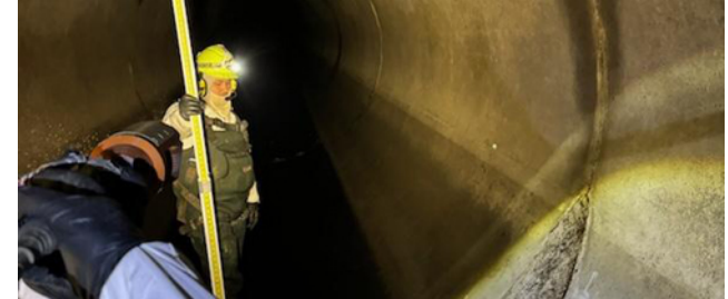
Emergency and Urgent Sewer Repair II
