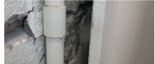
Structural Inspection and Structural Improvements
