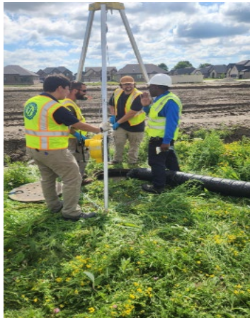
GLWA team members help lower a camera down into the sewer line
