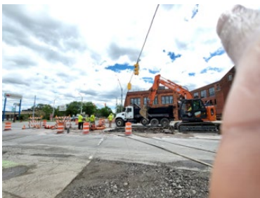
Work being performed at Stage 3 Michigan and Rosa Parks
