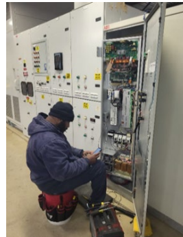
Marcus Henderson and Shane Clarke are here installing and wiring a new transformer to bring power to new equipment being installed in the cabinet at Imlay Station.
