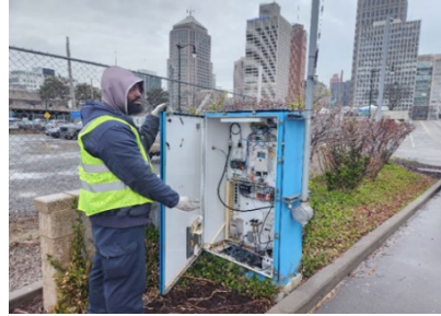
Backwater Gate #23, Control cabinet assessment
