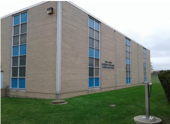
Figure 29. Newburgh Pump Station
