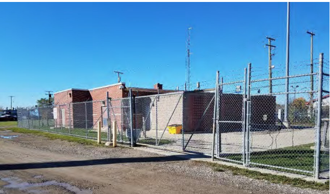
Figure 26: Michigan Avenue Pump Station
