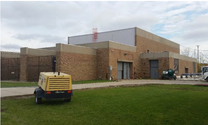
Figure 61. Northeast Pump Station
