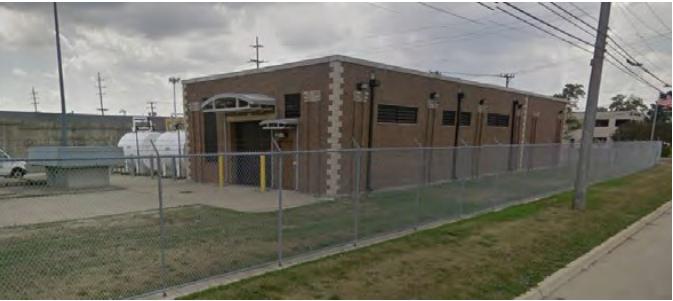
Figure 35. Schoolcraft Pump Station
