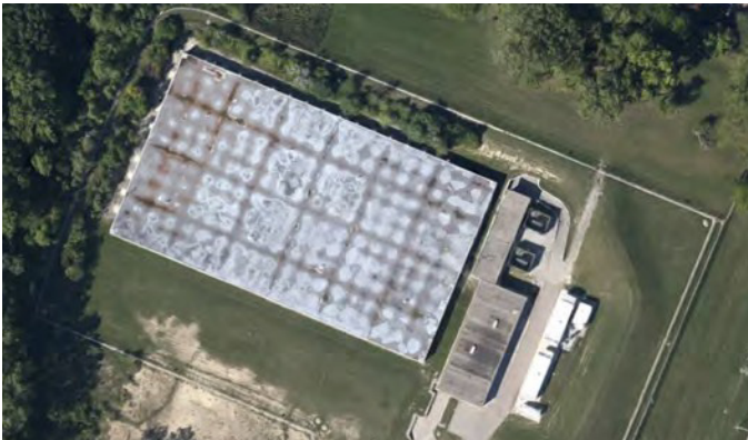
Figure 25. Franklin Pump Station
