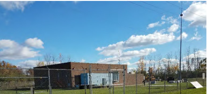
Figure 38. Ypsilanti Pump Station
