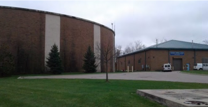
Figure 23: Haggerty Pump Station
