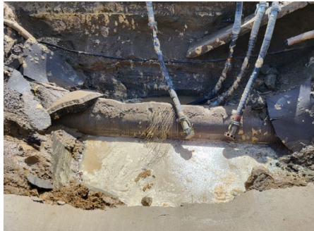
Broken 42-inch water main on 14 Mile Road in City of Novi
