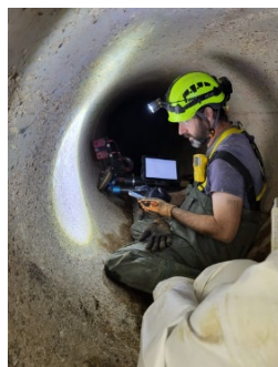
New 42-inch partially backfilled and inspection of existing 42-inch water main
