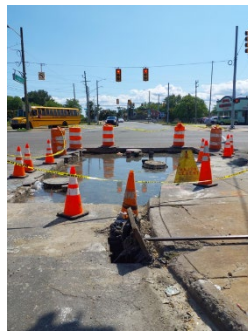
Investigating leak at Harper Avenue and Chalmers Street in City of Detroit
