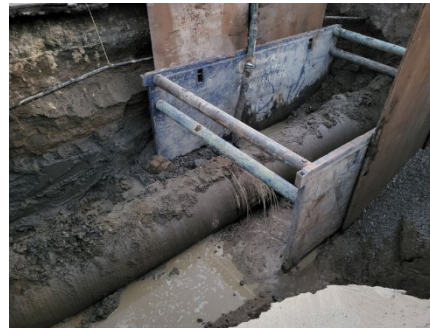
Broken 42-inch water main on 14 Mile Road in City of Novi
