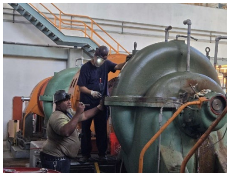
Removal of High Lift Pump No. 10 impeller
