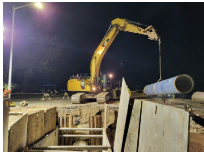
Installing new 42-inch steel water main
