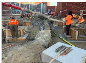
Main Canopy Storm Drain Lines
