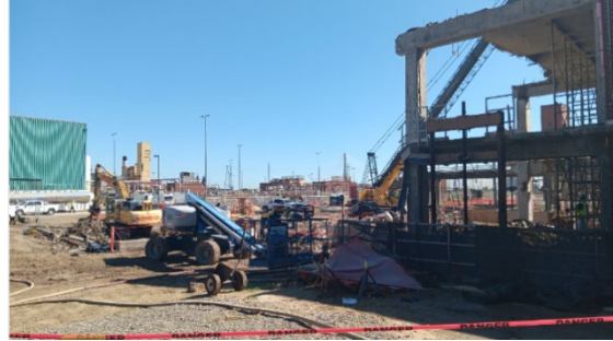
Screenings Building Demolition
