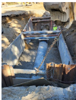
New 42-inch partially backfilled and inspection of existing 42-inch water main
