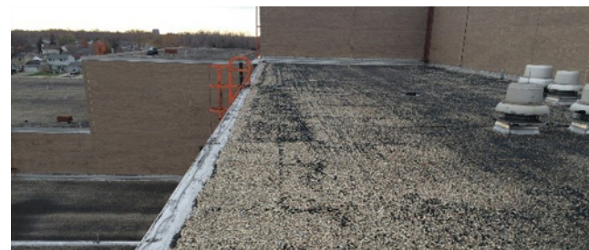
Lake Huron and Southwest Roof
