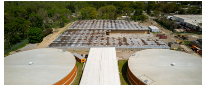
West Service Center Pumping Station
