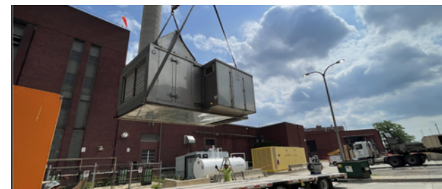
PS 1 Rack and Grit HVAC System Upgrade
