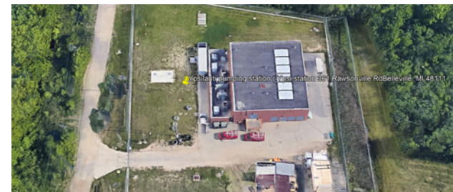
Ypsilanti Booster Pumping Station
