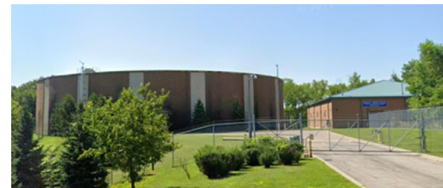
Imlay Pumping Station
