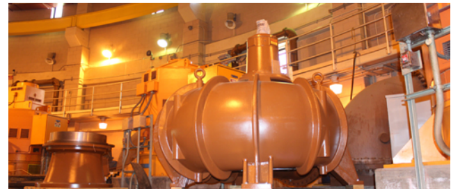
WRRF PS No. 2 Improvements Phase II
