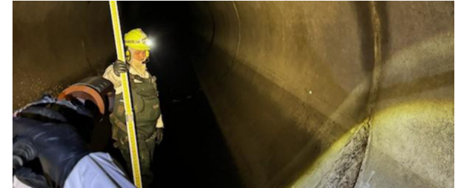
Emergency and Urgent Sewer Repair II
