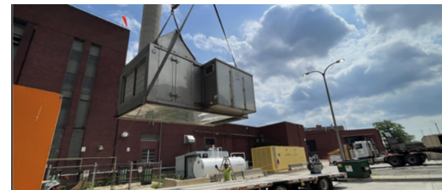
PS 1 Rack and Grit HVAC System Upgrade
