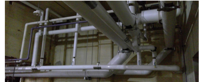
Condensate Return, and Compressed Air Piping
