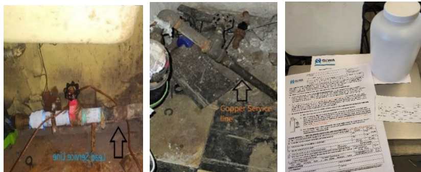
Pictured left to right: Lead service line, copper service line, and sampling kit
