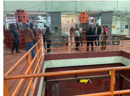
WWBP Work Group Members tour the Freud Pump Station
