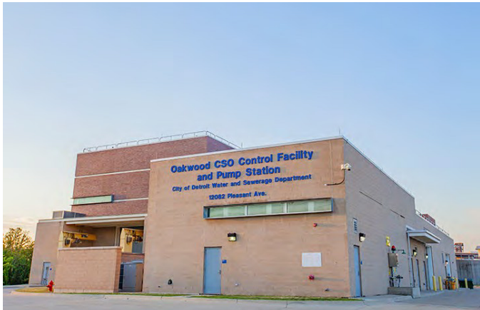
Figure 42. Oakwood CSO RTB
