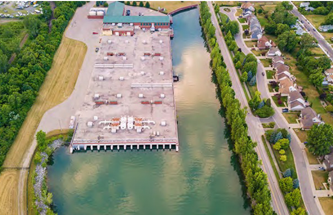
Figure 40. Conner Creek CSO RTB
