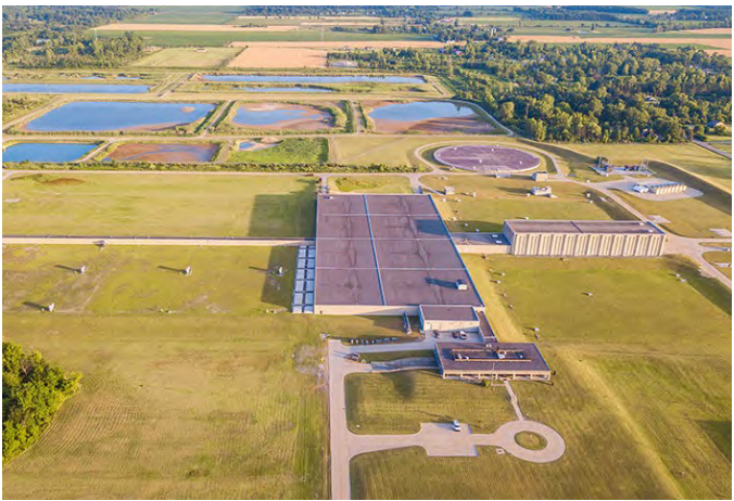
Figure 3. Lake Huron WTP
