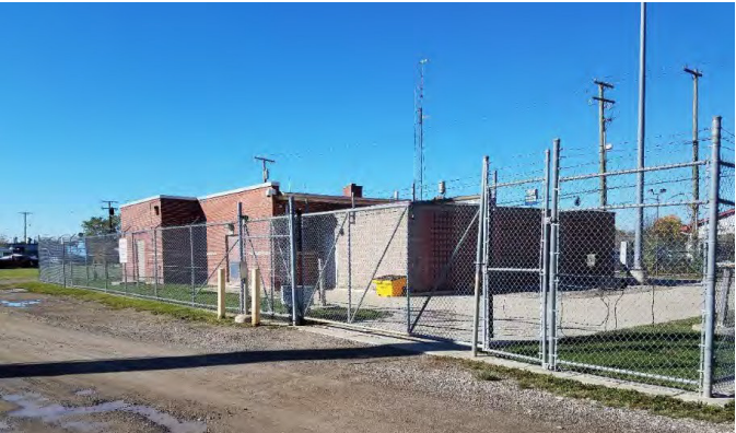
Figure 26: Michigan Avenue Pump Station
