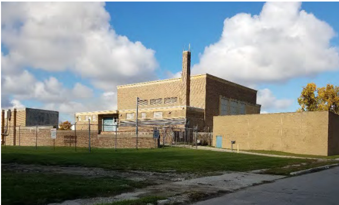
Figure 59. Freud Pump Station
