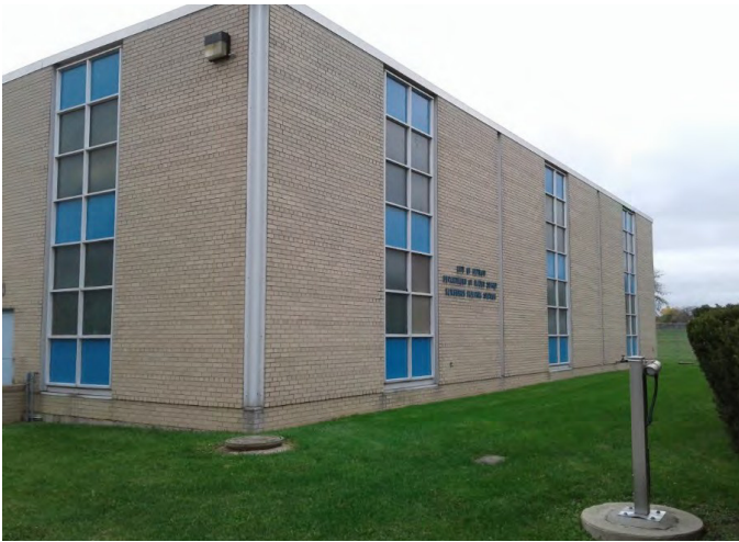
Figure 29. Newburgh Pump Station
