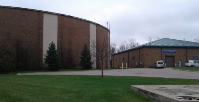
Figure 23: Haggerty Pump Station
