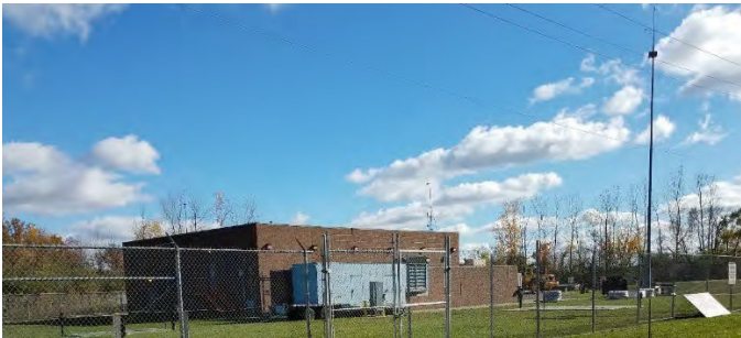
Figure 38. Ypsilanti Pump Station
