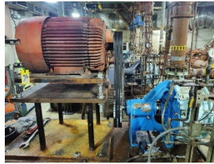
Right: Old pump-motor unit with liquid drive. Left: Liquid drive removed and pump-motor unit now direct drive.
