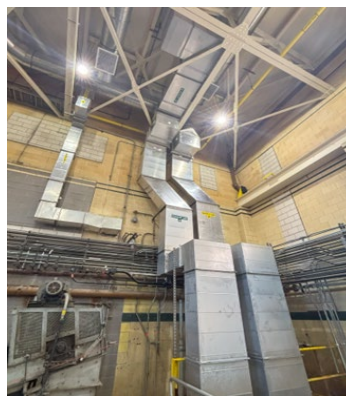
New Modified Duct Work at NE Wall
