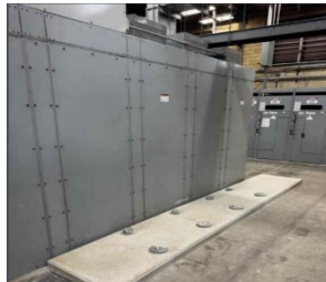
Housing Pads for Medium Volt MCC
