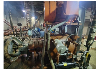
Right: Old pump-motor unit with liquid drive. Left: Liquid drive removed and pump-motor unit now direct drive.
