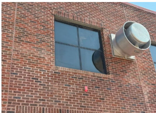
EF-1 Installation and Brick Repairs
