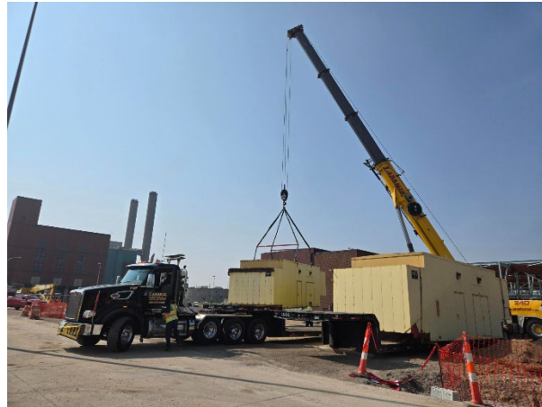
Removal of Generator D-1
