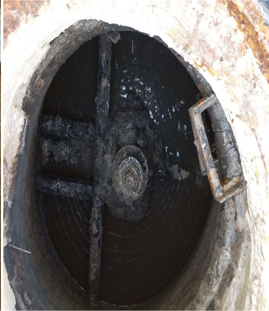
Operational Nut Rounded/Missing
