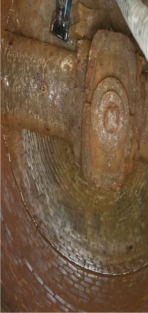
Operational Nut Rounded/Missing
