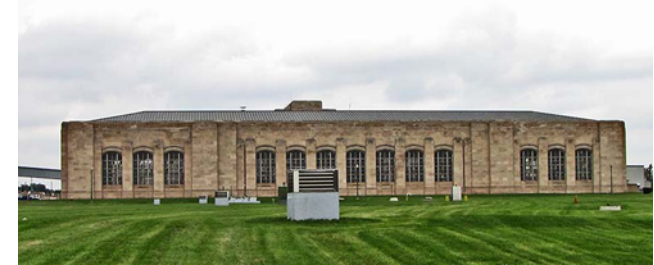
Administration Building Improvements
