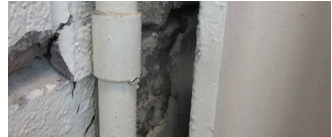
Structural Inspection and Structural Improvements
