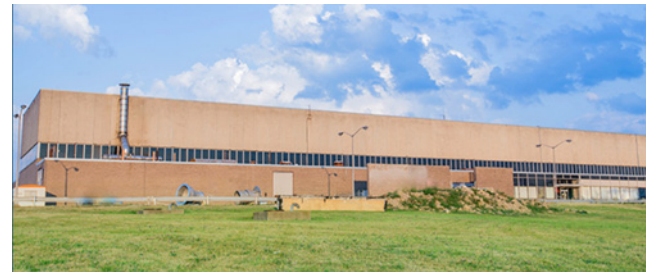
Southwest Water Treatment Plant
