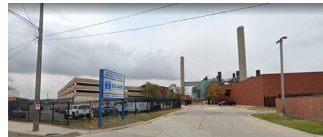
WRRF Front Entrance Rehabilitation
