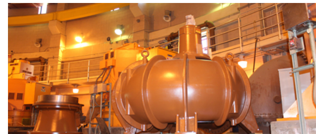
WRRF PS No. 2 Improvements Phase II
