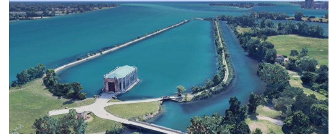
Belle Isle Seawall
