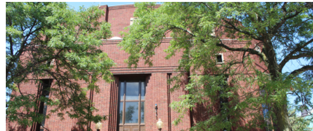
WRRF PS No. 1 Improvements
