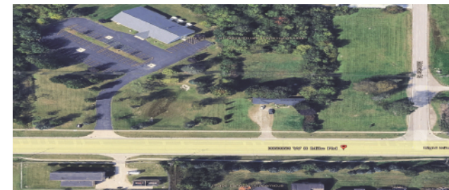
Newburgh Road Booster Pumping Station
