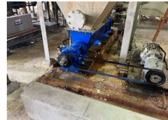
The old scum hopper pump removed (l), and the new pump installed (r)
