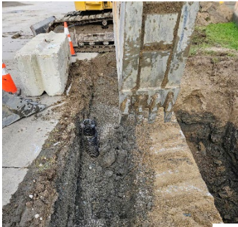
TWAS Mechanical Cleaning Excavation
