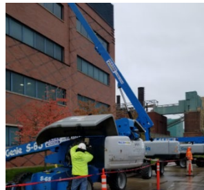
Window caulking replacement at the NAB
