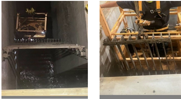
West wet well bar rack removal at Oakwood CSO Pumping Station
