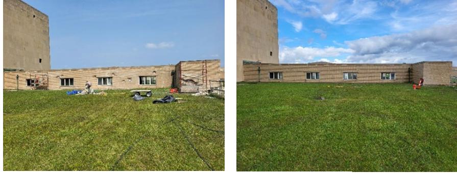
Brick removal and replacement
