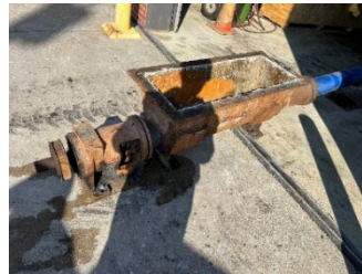
The old scum hopper pump removed (l), and the new pump installed (r)
