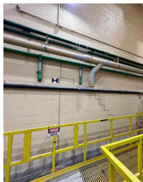
Wall repairs at Puritan Fenkell Facility
