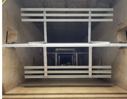
New flocculator shafts and paddles
