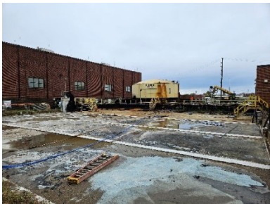
Pickle Liquor Foundation Demolished
