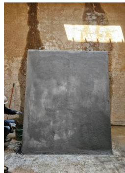
New baffle wall for inlet improvements
