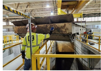
Screen # 4 is being rehabilitated
