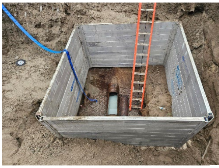
TWAS Line Prepared for Mechanical Cleaning
