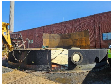
Chemical Building Tank 1 Demolition
