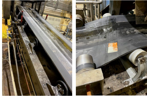
The new vulcanized belt installed at Grit Cross-conveyor 1
