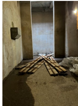
Demolished inlet controls
