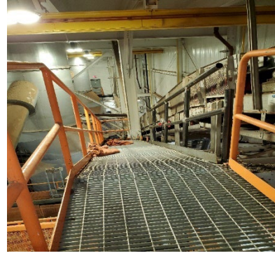
New handrails at conveyor H
