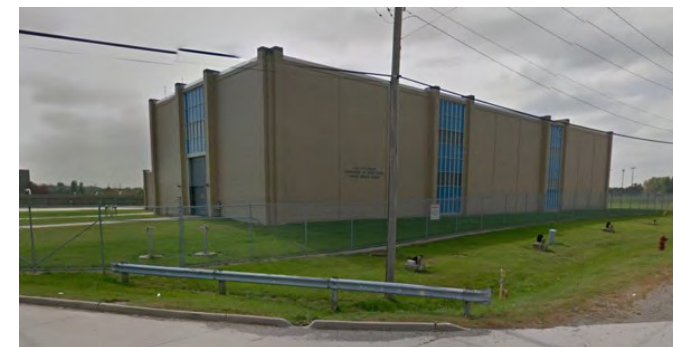
Figure 31. North Service Center
