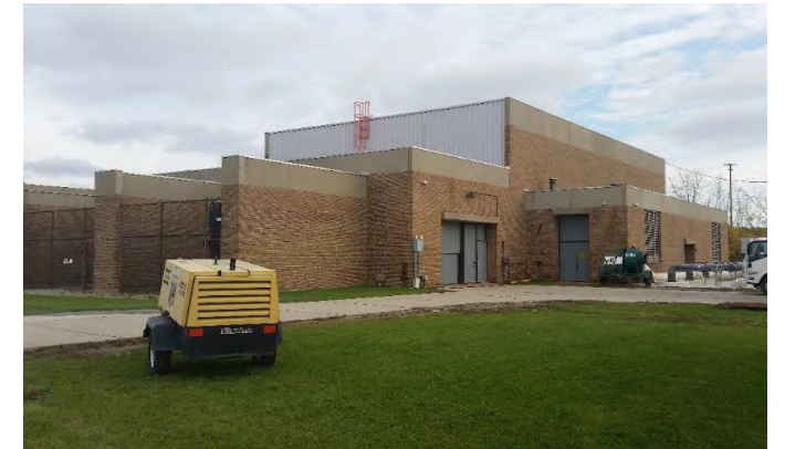
Figure 61. Northeast Pump Station
