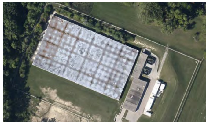
Figure 25. Franklin Pump Station
