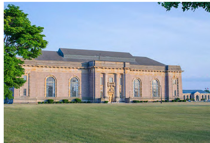
Figure 10. Water Works Park WTP
