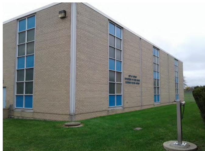
Figure 29. Newburgh Pump Station
