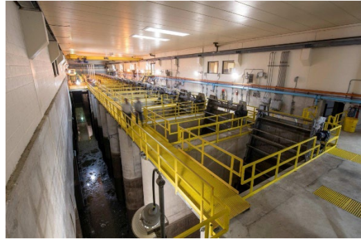
The GWK retention treatment basin serves 14 municipalities in southeast Oakland County capturing and treating combined stormwater and sanitary flow during storms
