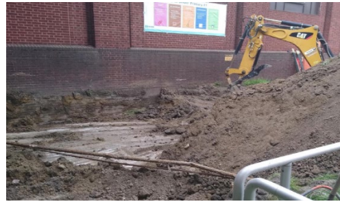
Excavation for a New Electrical
