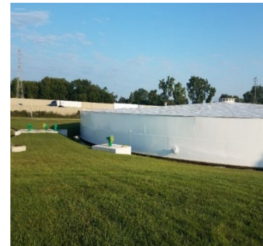
Reservoir #1 Southwest WTP freshly painted
