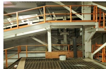
Location of the new access platform
