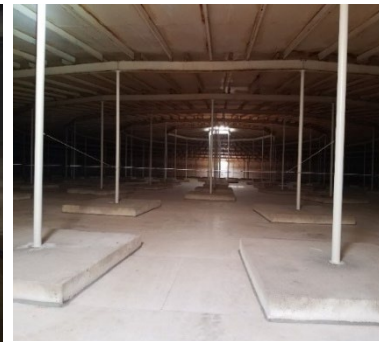
Interior of Springwells WTP Reservoir #1 finalized for inspection
