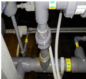
Ferric Chloride pipe break at union connection Pipe support anchor failure
