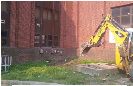
Existing Cooling Unit Pad Removal
