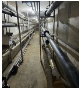
Work at Service Tunnel
