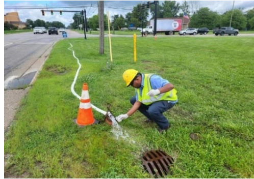
36-inch transmission main
