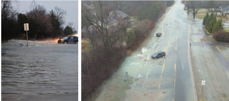
14 Mile Road 48-inch water main break
