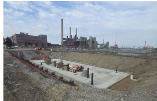
New concrete foundation over West effluent channel
