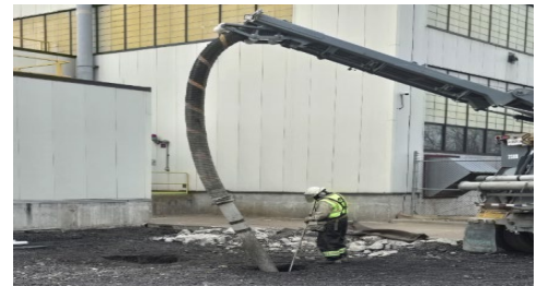
Contractor using hydroexcavation to install vibration monitors near Dechlorination facility
