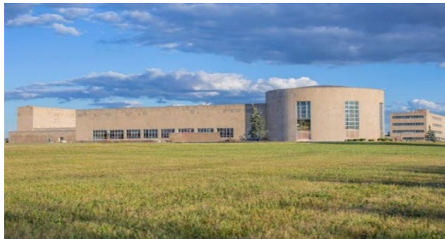
Northeast Water Treatment Plant
