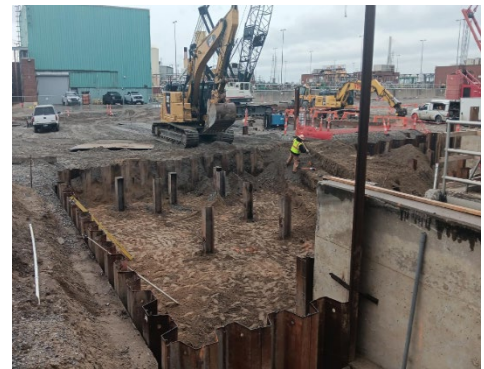
Earth retention sheet piles on north side of PS2
