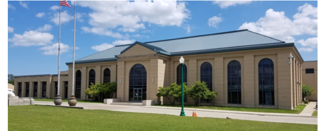
As-Needed Geotechnical and Related Engineering Services
