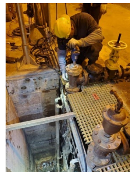
Maintenance team member installing new sump pumps
