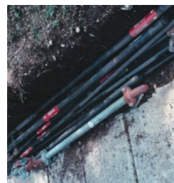
CO2 fire suppression system piping after being removed
