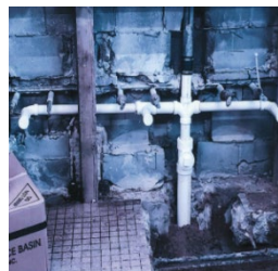
A section of new plumbing in the Warehouse and the in-progress renovation of the bathroom
