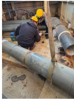
Maintenance team members measuring fluoride line to insert alternate feed
