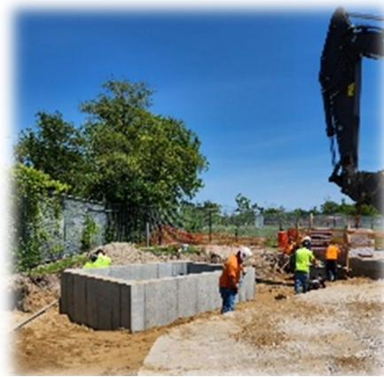
Northwest reservoir isolation valve man way
