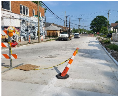
Concrete pavement restoration on Beard Street, and restoration at the intersection of Beard Street and Rowan Street
