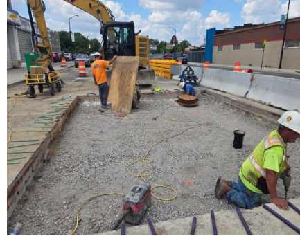
Leaking 42-inch watermain, contractors installed repair clamp and roadway
