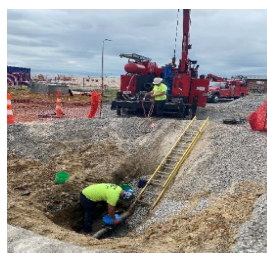
Line stop installation by Watertan
