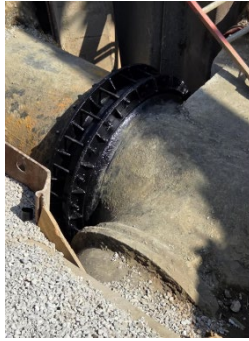
Leaking 42-inch watermain, contractors installed repair clamp and roadway
