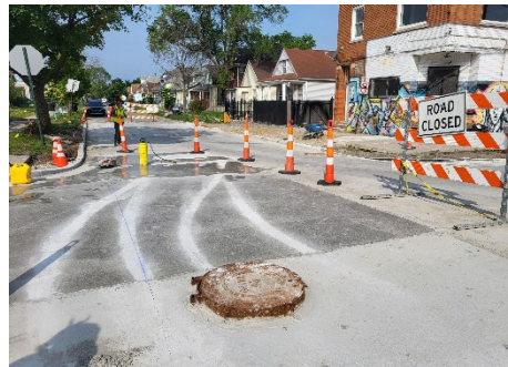
Concrete pavement restoration on Beard Street, and restoration at the intersection of Beard Street and Rowan Street
