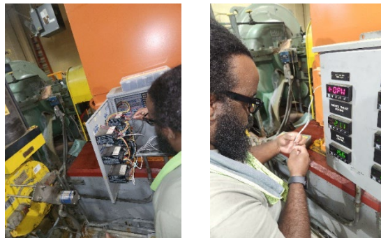
Josh Walker working at the Ypsilanti Station repairing the wiring for one of the temperature probes for the line No. 2 motor
