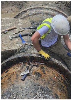
Leaking 42-inch watermain, contractors installed repair clamp and roadway
