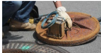
Installation of a SmartCover instrument
