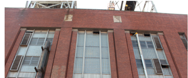
WRRF Roof Replacement for Multiple Facilities Program
