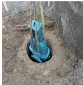
New Isolation valve being lowered into place
