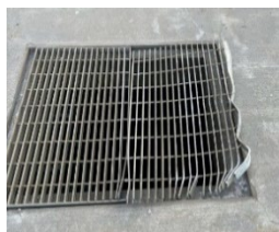
Damaged grating
