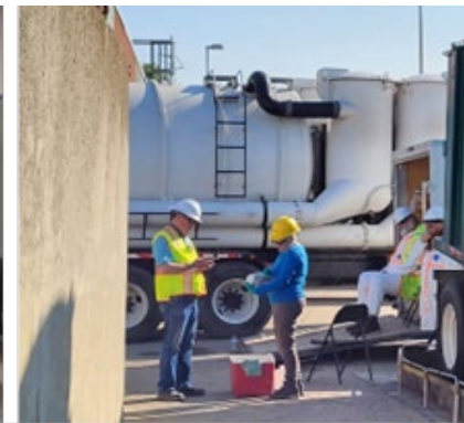
Chemist Natalia Chevtchenko (right) during sample collection of the spent washing solution after removal of vivianite deposits from a sludge line.
