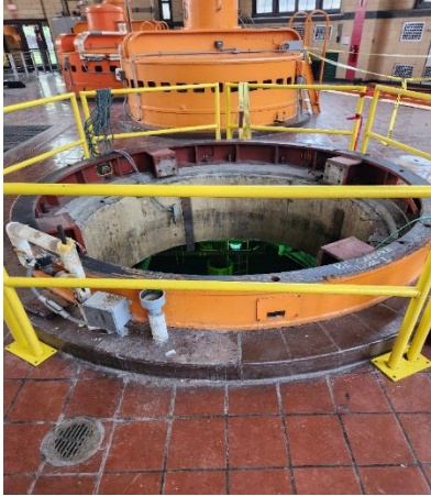
View of the removed motor and shafting from the Pump Station 1 motor floor and the new POA in the process of being moved into Pump Station 1
