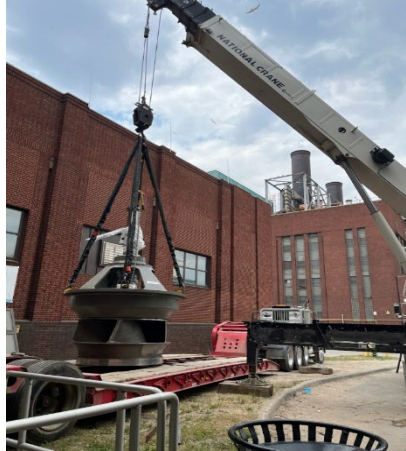
View of the removed motor and shafting from the Pump Station 1 motor floor and the new POA in the process of being moved into Pump Station 1
