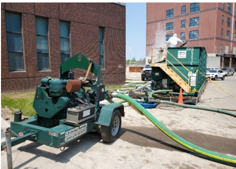
Chemical Cleaning of permanent TWAS line
