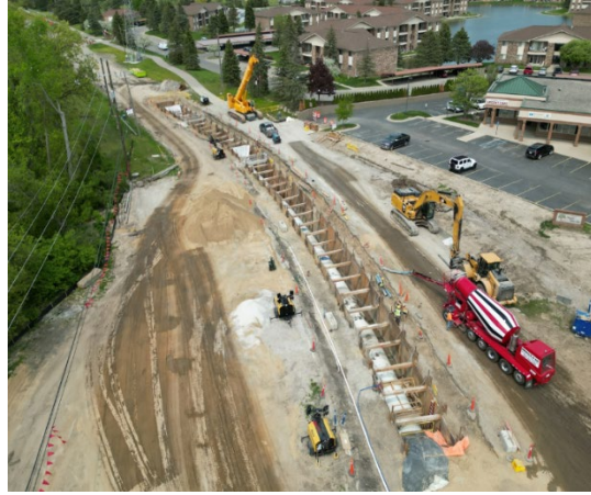
96-inch WTM installation on Dequindre Rd. north of 23-mile intersection
