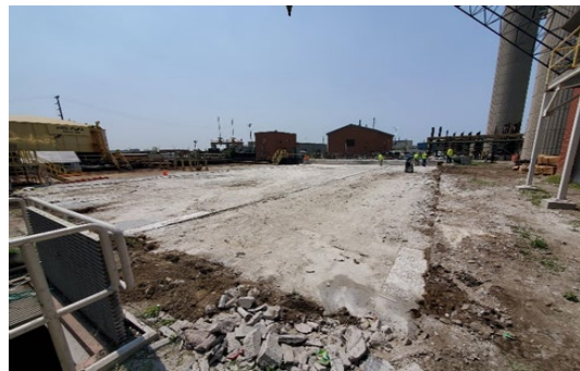
Three Ferric Chloride Tanks Removed
