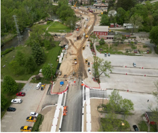
Avon Road restoration activities after water transmission main installation
