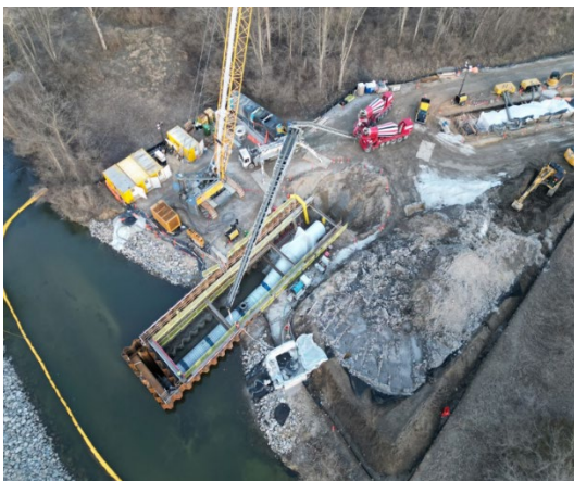
Cofferdam on south side of Clinton River
