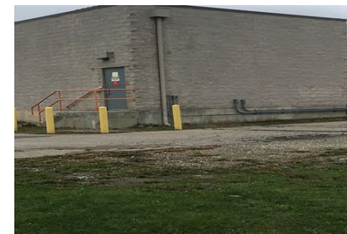
Figure 20. Adams Road Pump Station
