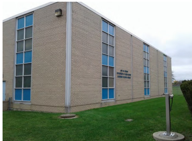
Figure 29. Newburgh Pump Station
