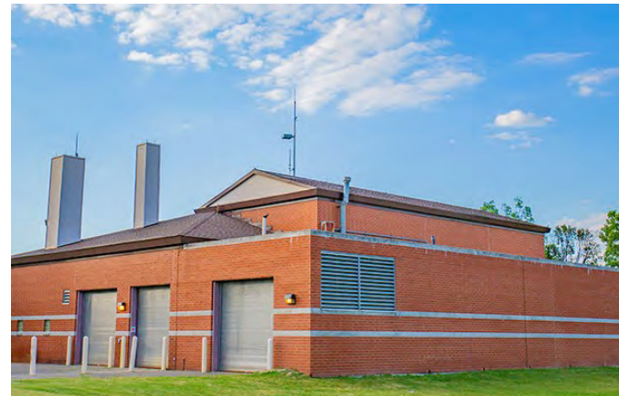
Figure 43. Puritan-Fenkell CSO RTB
