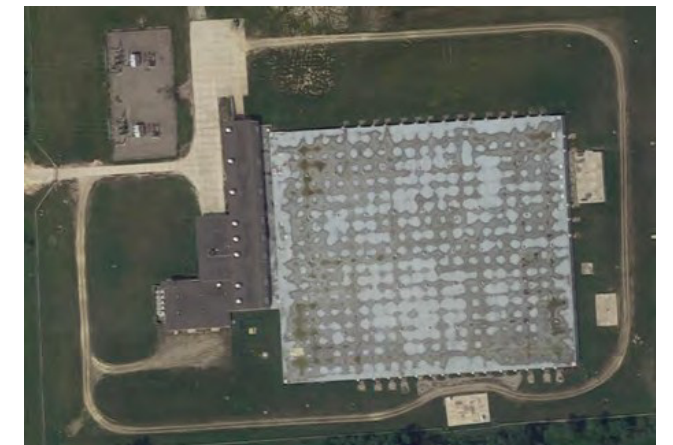
Figure 28. Imlay Pump Station
