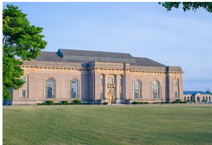
Figure 10. Water Works Park WTP
