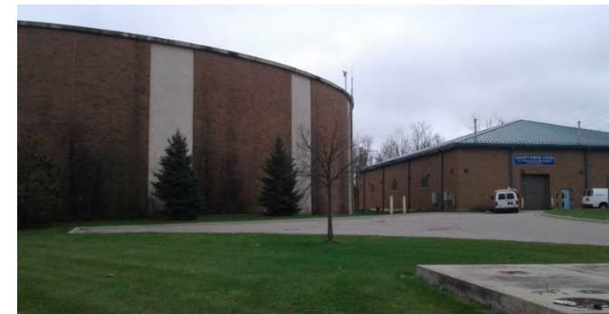
Figure 23: Haggerty Pump Station
