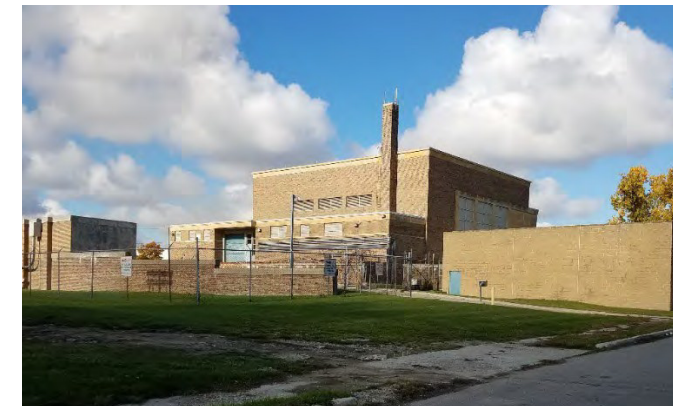
Figure 59. Freud Pump Station
