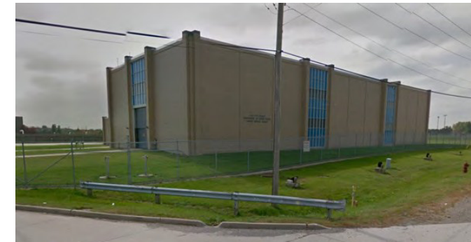
Figure 31. North Service Center
