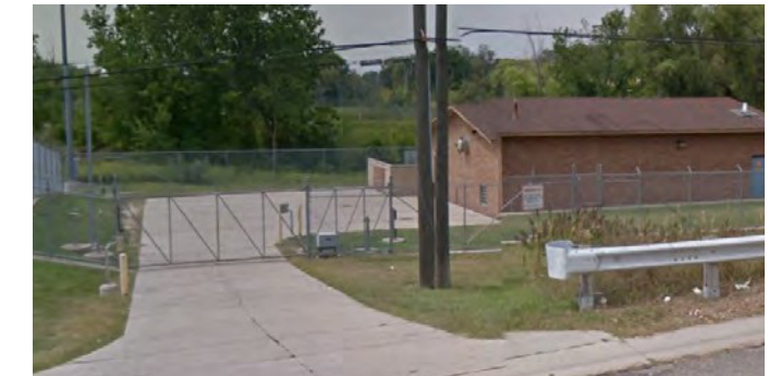
Figure 32. Orion Pump Station
