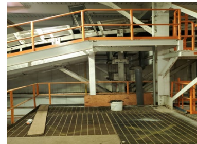
Location of the new access platform
