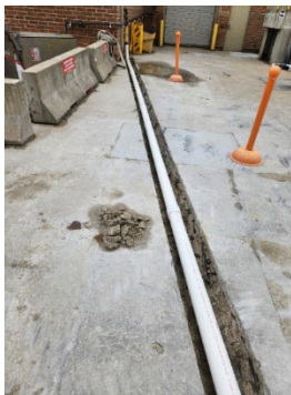
New natural gas line installed inside of PVC pipe
