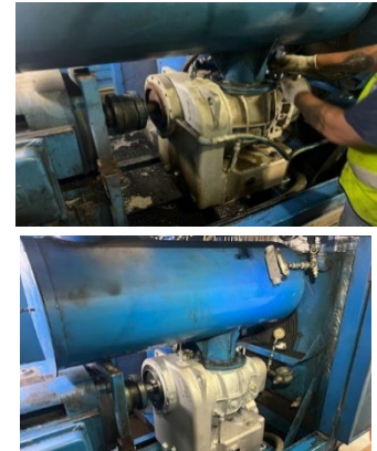
The old blower being removed, and the new blower installed
