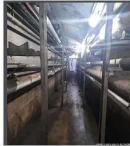
Existing Electrical Conduits Removal at Service Tunnel
