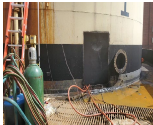
Power Washing to Remove Rubber
