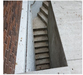
Task 2J-01 Upper Wet Well Stairwell
