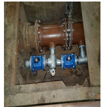
Task 70 SST No. 1 and 3 Equalization Valve
