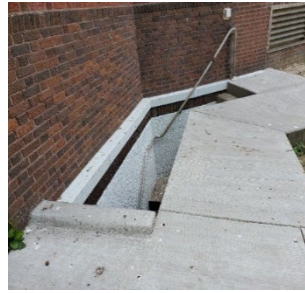
Task J2-01 Upper Wet Well Stairwell
