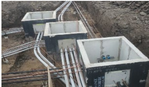
Duct bank installation near venturi meter M-06
