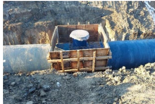
Air release valve foundation formwork
