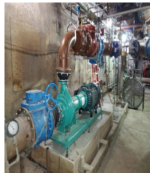
Task 70 Complex A Gallery SFP-2 Pump Replacement
