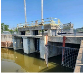
Shunt bypass emergency gates at Hubbell-Southfield
