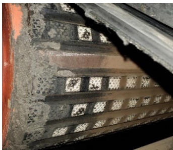
Failed Conveyor Drive Pulley
