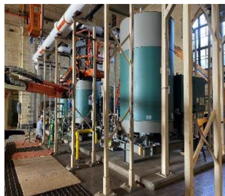
Aerial view of installation of 3 new steam
