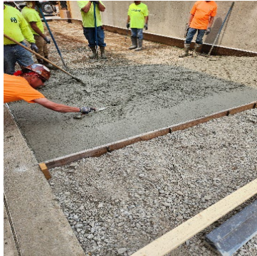
New Concrete West of Chemical Building
