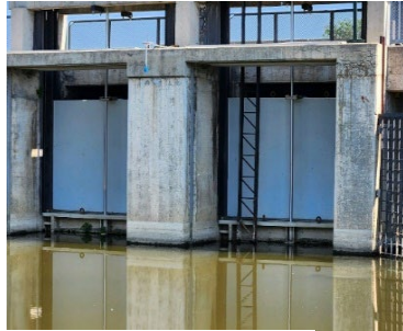
Shunt bypass emergency gates at Hubbell-Southfield
