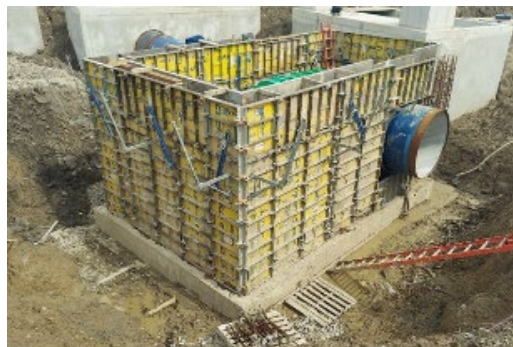
Formwork for valve vault V-06
