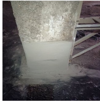
Spall repairs at HS Basin
