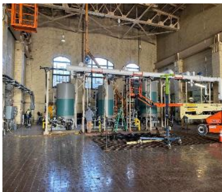
Installation of three new steam generators in progress
