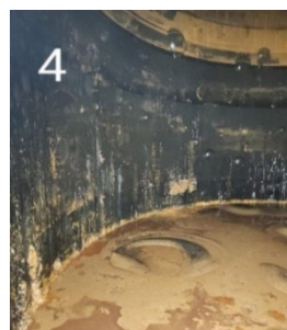
Tank #2 lining - Bubbled gasket lining
