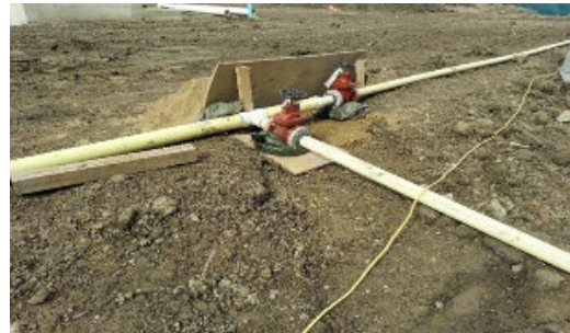
4-inch temporary main for pressure testing
