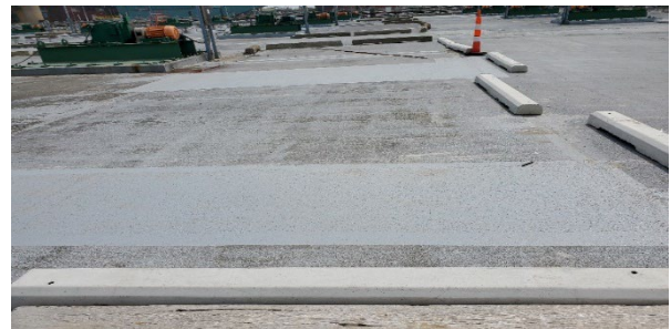
Newly installed planks under task J2-05
