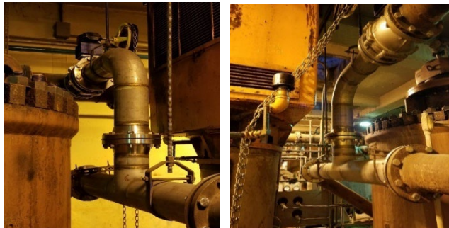
The new backwash line installed for the #7 SFE pump
