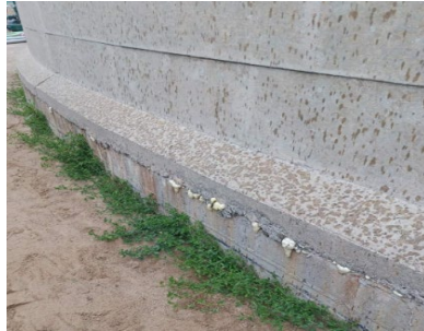
STT-14 Leak Repairs
