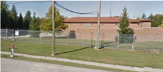
Figure 33. Rochester Pump Station
