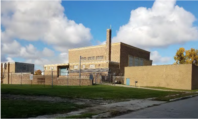
Figure 59. Freud Pump Station
