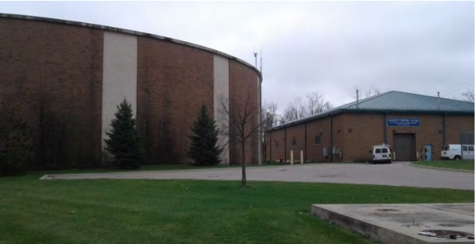
Figure 23: Haggerty Pump Station
