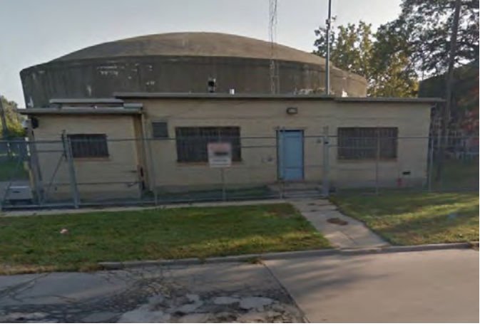
Figure 22. Electric Avenue Pump Station
