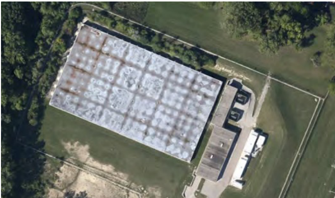
Figure 25. Franklin Pump Station
