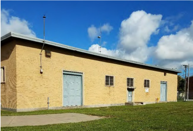
Figure 21. Eastside Pump Station
