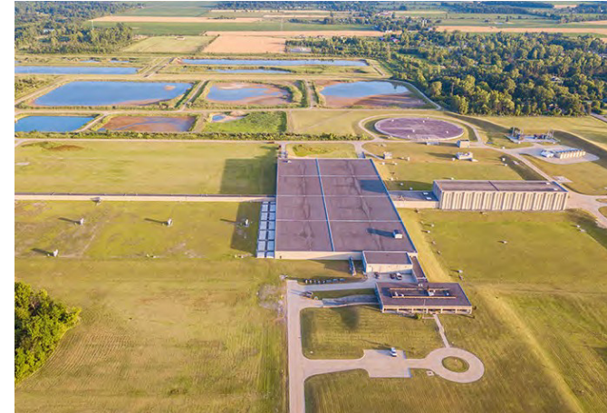
Figure 3. Lake Huron WTP
