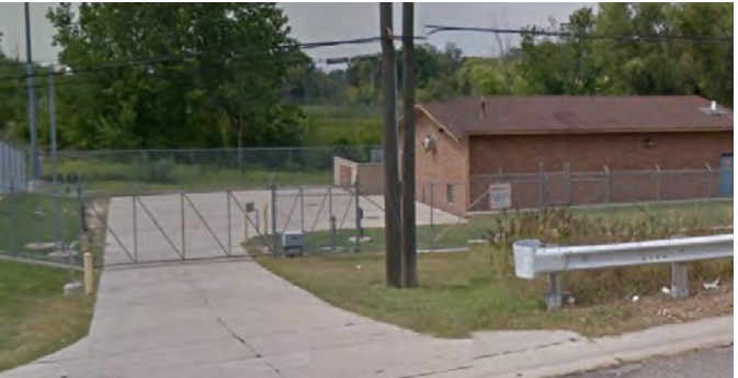
Figure 32. Orion Pump Station
