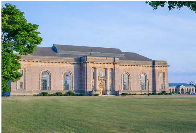
Figure 10. Water Works Park WTP
