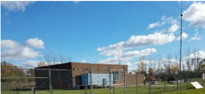
Figure 38. Ypsilanti Pump Station
