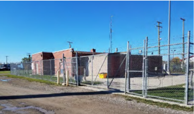
Figure 26: Michigan Avenue Pump Station
