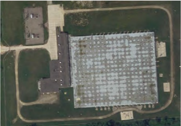
Figure 28. Imlay Pump Station
