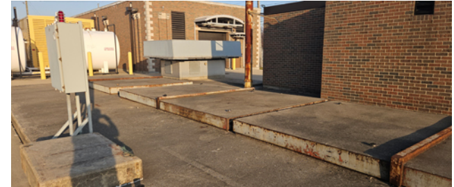
Schoolcraft Pumping Station
