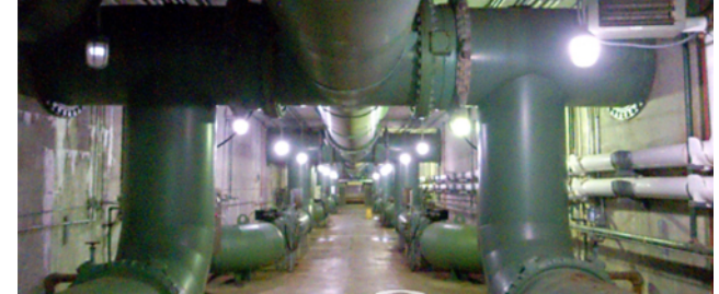
WTP Filtration Improvement
