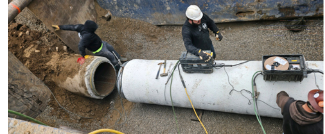
Transmission System Valve
