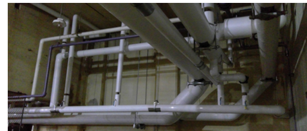
Condensate Return, and Compressed Air Piping
