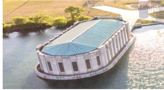
Belle Isle Intake
