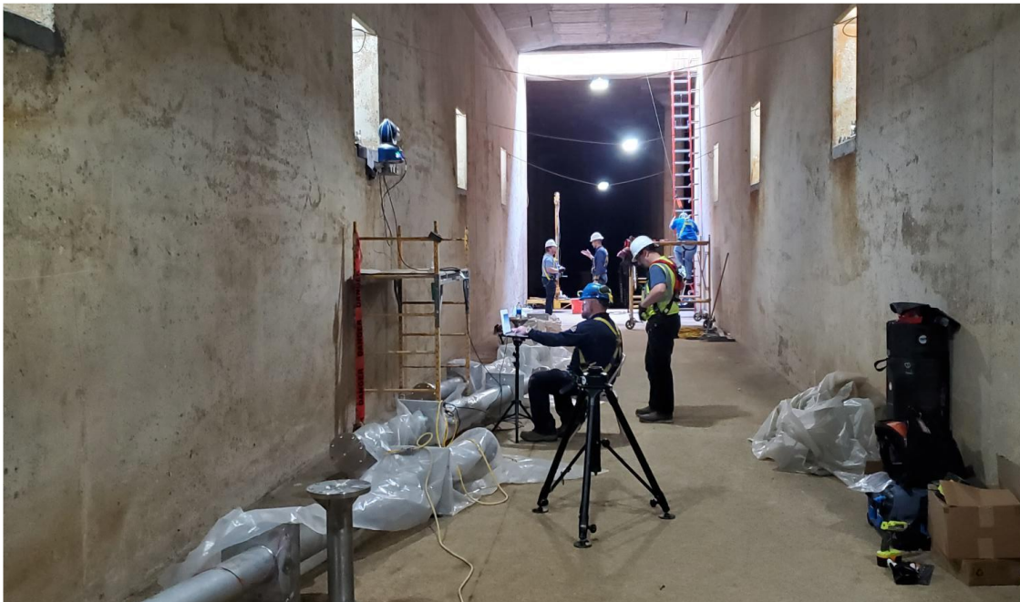
Flocculator Alignment
