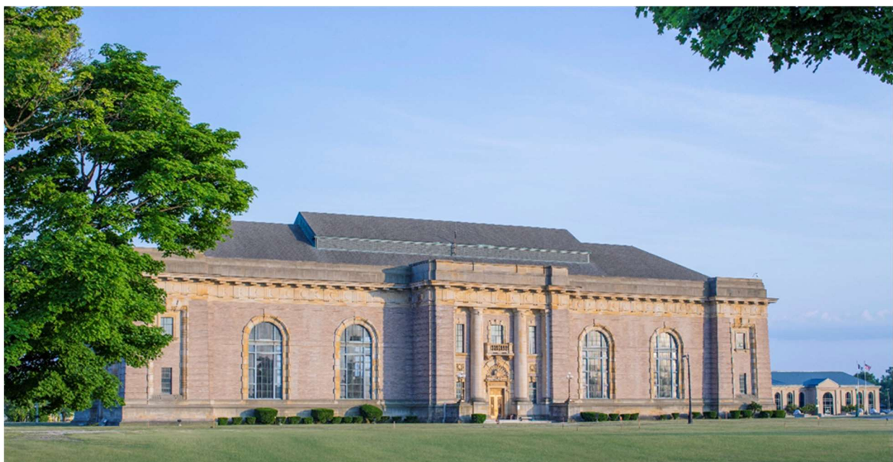
GLWA Water Works Park Water Treatment Facility
