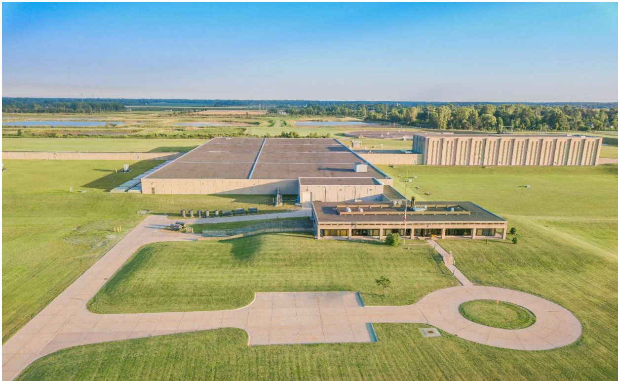
GLWA Lake Huron Water Treatment Facility
