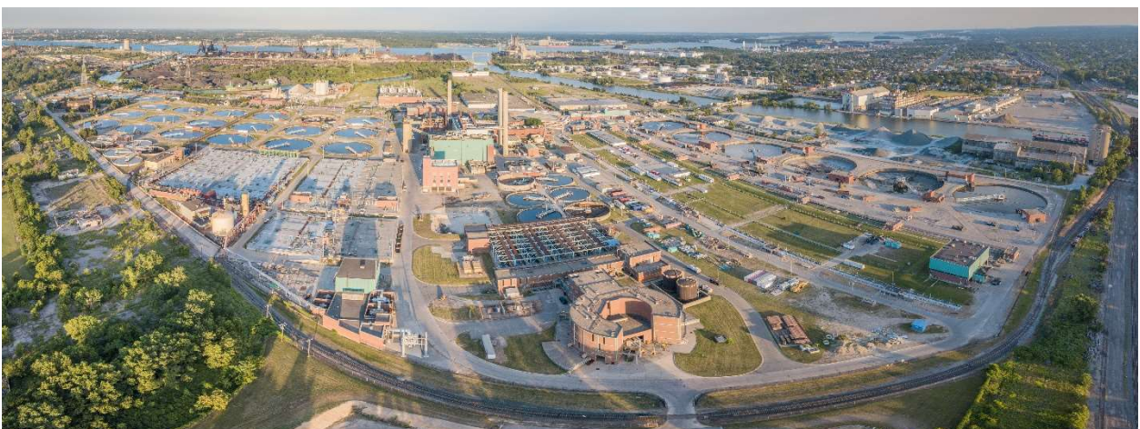
GLWA Water Resource Recovery Facility
