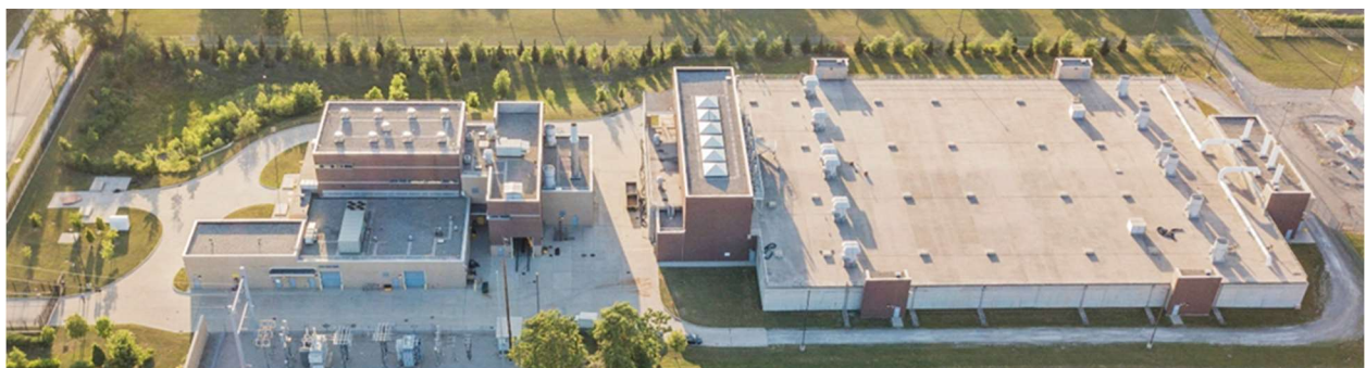
GLWA Hubbell-Southfield Facility
