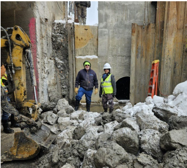
Nearly Completed Fox-Creek to DRI Flushing Structure
