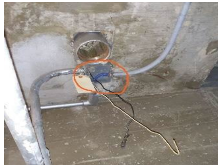
Safety violations found at Michigan Avenue Station (exposed electrical wires)
