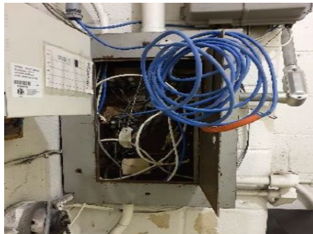
Safety violations found at Michigan Avenue Station (exposed electrical wires)
