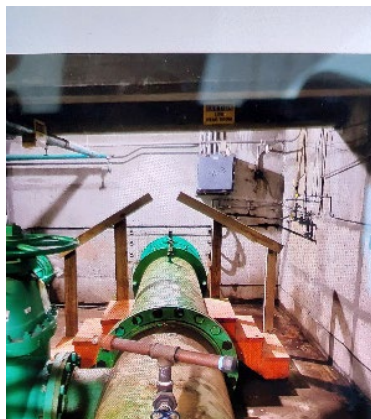
Rebuilt stairs and platforms at Haggerty Station
