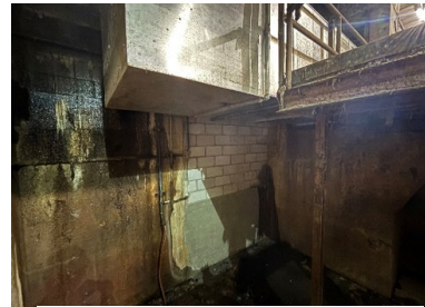
Block wall in Conveyor Tunnel
