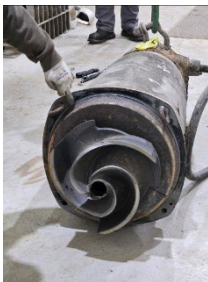
GLWA Maintenance Team replacing the impeller after training, shown in
