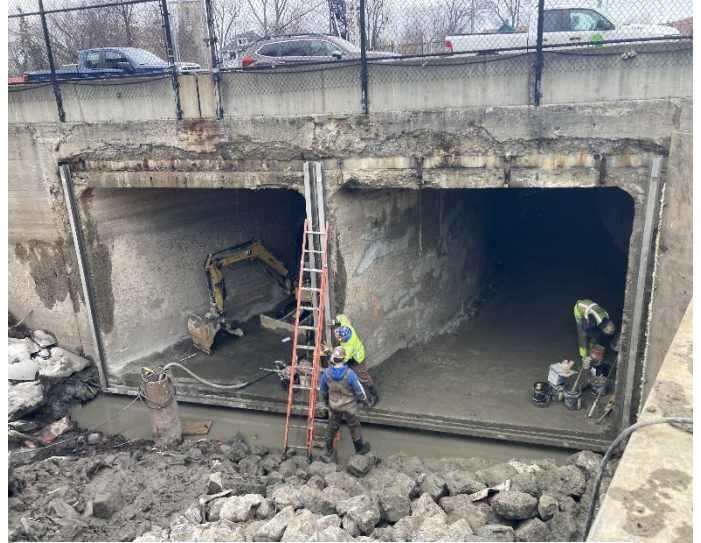
Cleaned B-01 Barrel Outlets at Fox Creek
