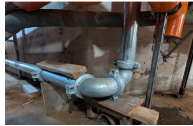
Potable water line installation
