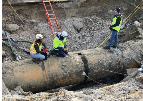
HDR and GLWA team members performing investigation on the 54" main
