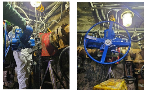
Dewatering Team working on the MOV-123 valve
