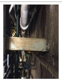
Photo 2: Failed Concrete Column in Administration Building Basement
