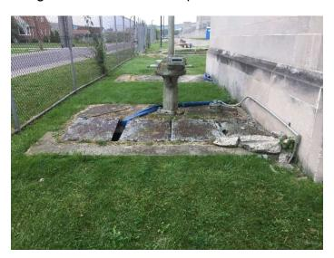
Photo 3: Deteriorated Concrete Slabs and Hatches at Drain Pump House
