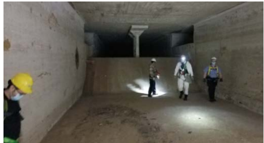
Plant staff inspecting settled water conduit in 1930 Filter Plant
