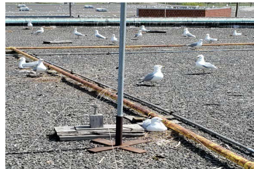
Seagulls on WRRF building roof
