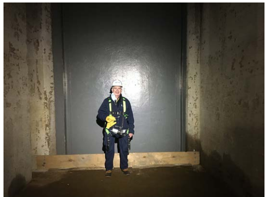
Lab Team Leader Andrew Ross standing in front of a new basin influent gate
