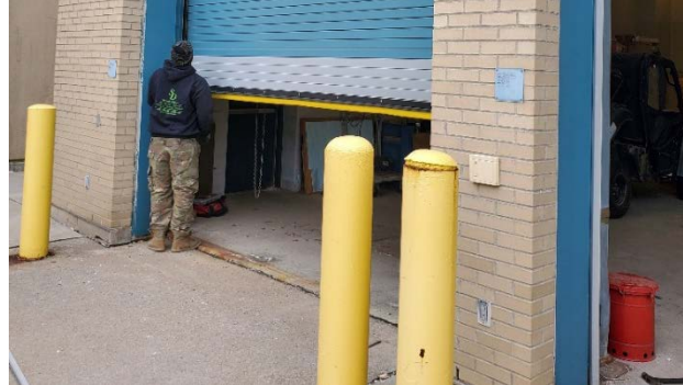
Bottom Slats and Safety Edge Replaced
