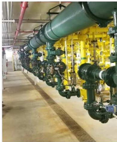
Sulphur Dioxide Injectors
