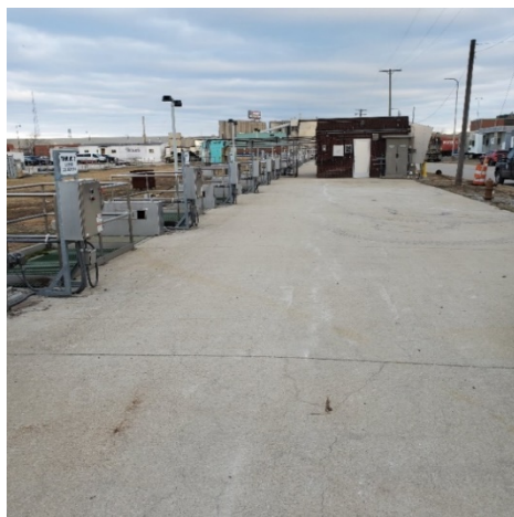
Clarifier drives, disconnect boxes and Drive covers (Typical clarifiers 1 – 12
