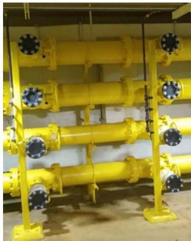
Pipelines for Sulphur Dioxide Solution water
