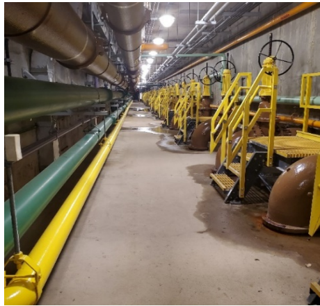
Stair platforms. Upper and lower sludge pipe headers
