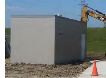
New staircase well access to Tunnel
