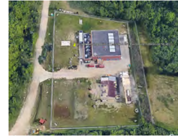
Existing Ypsi station
