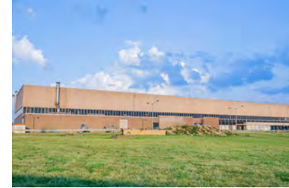
SW SCADA System Upgrade
