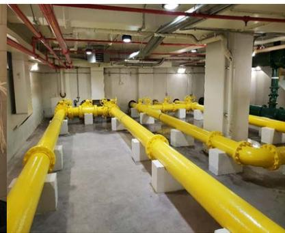
Painted chlorine solution feed lines with new LED lighting in basement pipe
